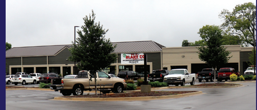
New H.C. Blake building on North Parkway
